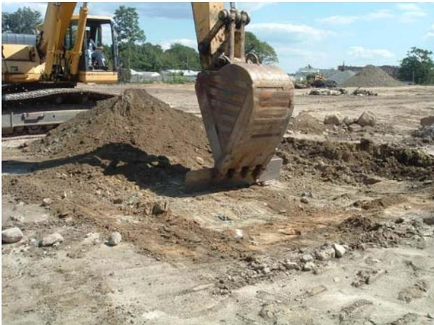
Scraping of surficial soil impacted by lead at ABC Auto
